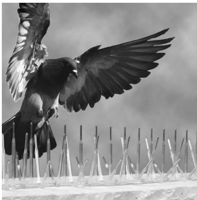
Bird spikes being used to prevent roosting.
